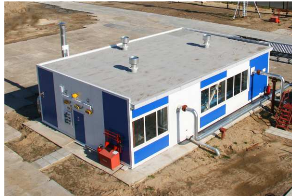
2010 - Prefabricated building of SIKN for Crude Oil Acceptance and Delivery Station of Oil Refinery in the village of Semiluzhki, Tomsk Oblast, OOO Tomskneftepererabotka
