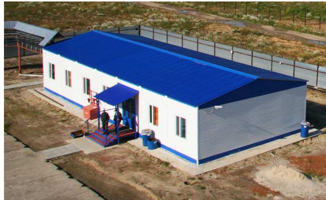
2010 - Administrative and on-site quarters for Crude Oil Acceptance and Delivery Station of Oil Refinery in the village of Semiluzhki, Tomsk Oblast, OOO Tomskneftepererabotka
