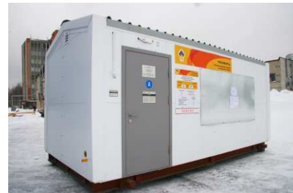
2009 - Prefabricated building for control room of MPS at Katangli oilfield OOO RN-Sakhalinmorneftegas, OAO NK Rosneft
