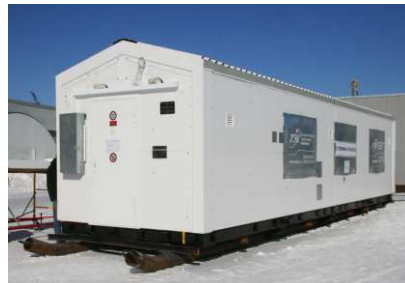
2009 - Prefabricated building for SIKN at Katangli oilfield OOO RN-Sakhalinmorneftegas, OAO NK Rosneft
