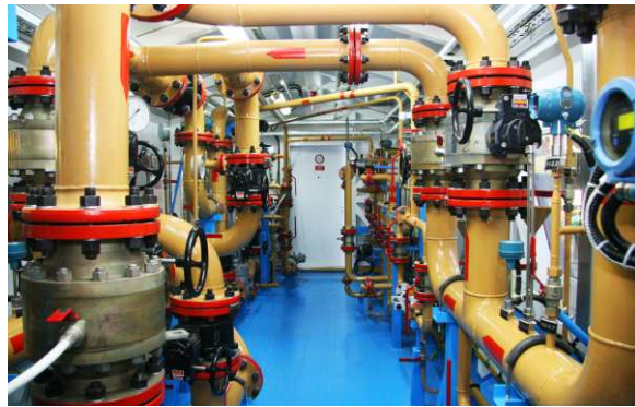
2009 - SIKNS for Odoptu-more oilfield, OOO RN-Sakhalinmorneftegas, OAO NK Rosneft. General View
